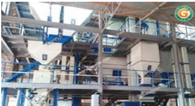
A well designed Feed Mixing Unit
