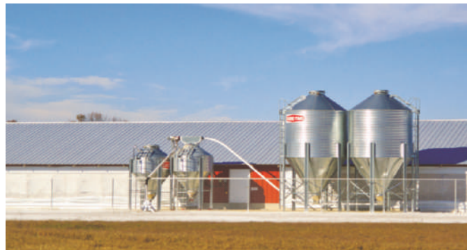
Feed Silo's outside the Poultry house with connecting Auger's
