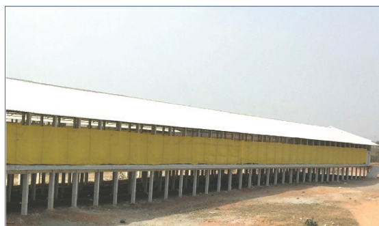
Figure 4. Lowering the curtain at the top creates better ventilation.
